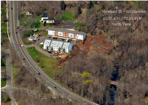
Landslide in Middletown
