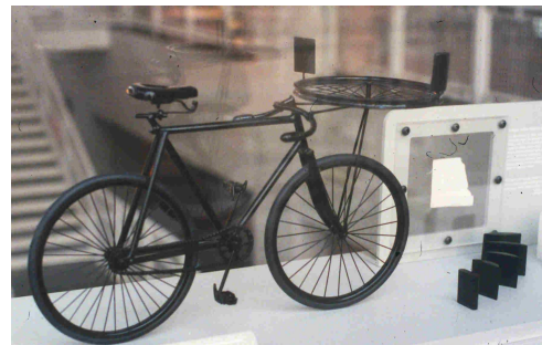
Above, a bicycle modified with a force balance and used by the Wrights to test airfoils, a converse wind tunnel. Below: A replica of a Wright wind tunnel on display at the General Thomas Stafford Aerospace Museum.
